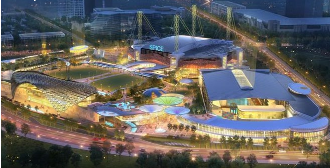
Subterranean Penang International Conference & Exhibition Centre
